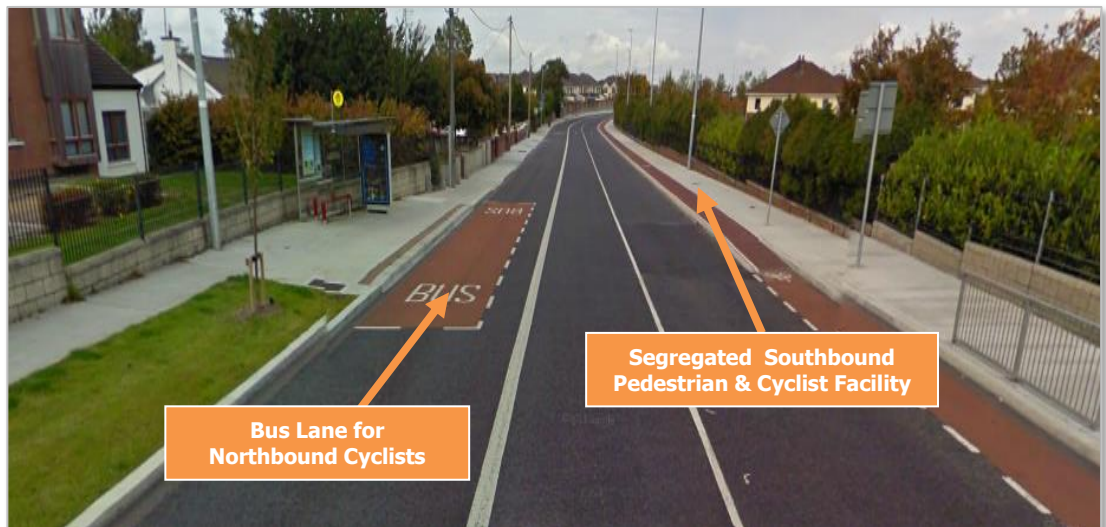
Figure 2.9: Cycling Facilities on Ballycullen Road
