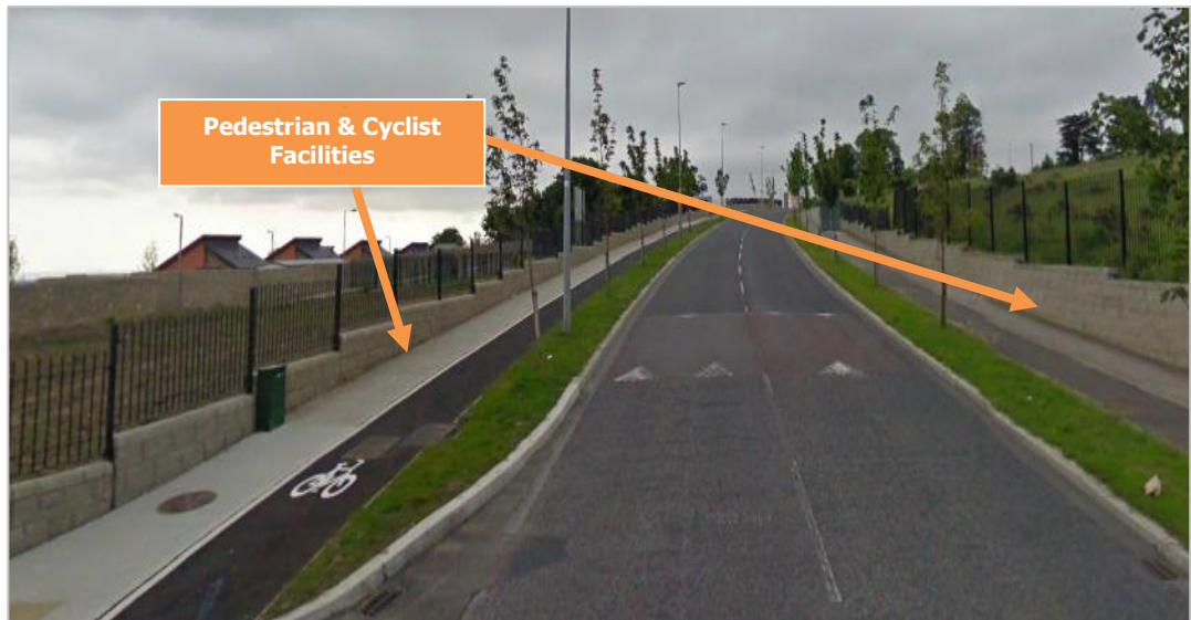
Figure 2.8: Stocking Avenue Looking East
